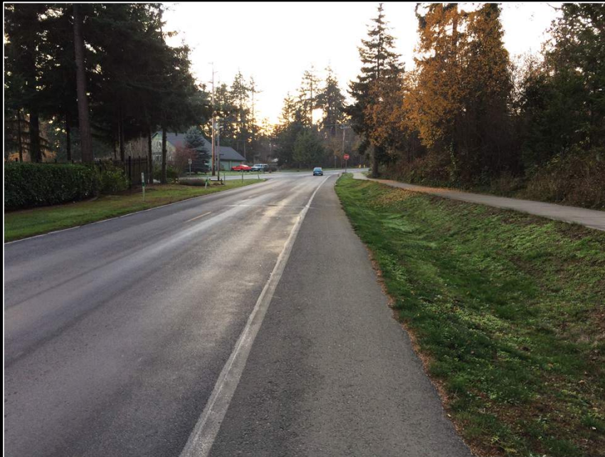
Discovery Road – Road side Swale
