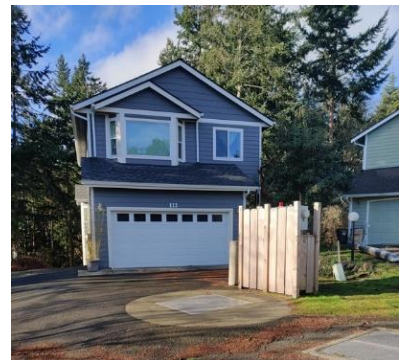
Island Vista Lift Station
