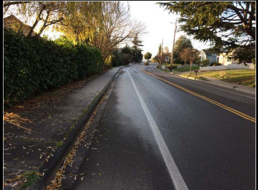
F Street – Curb and Gutter
