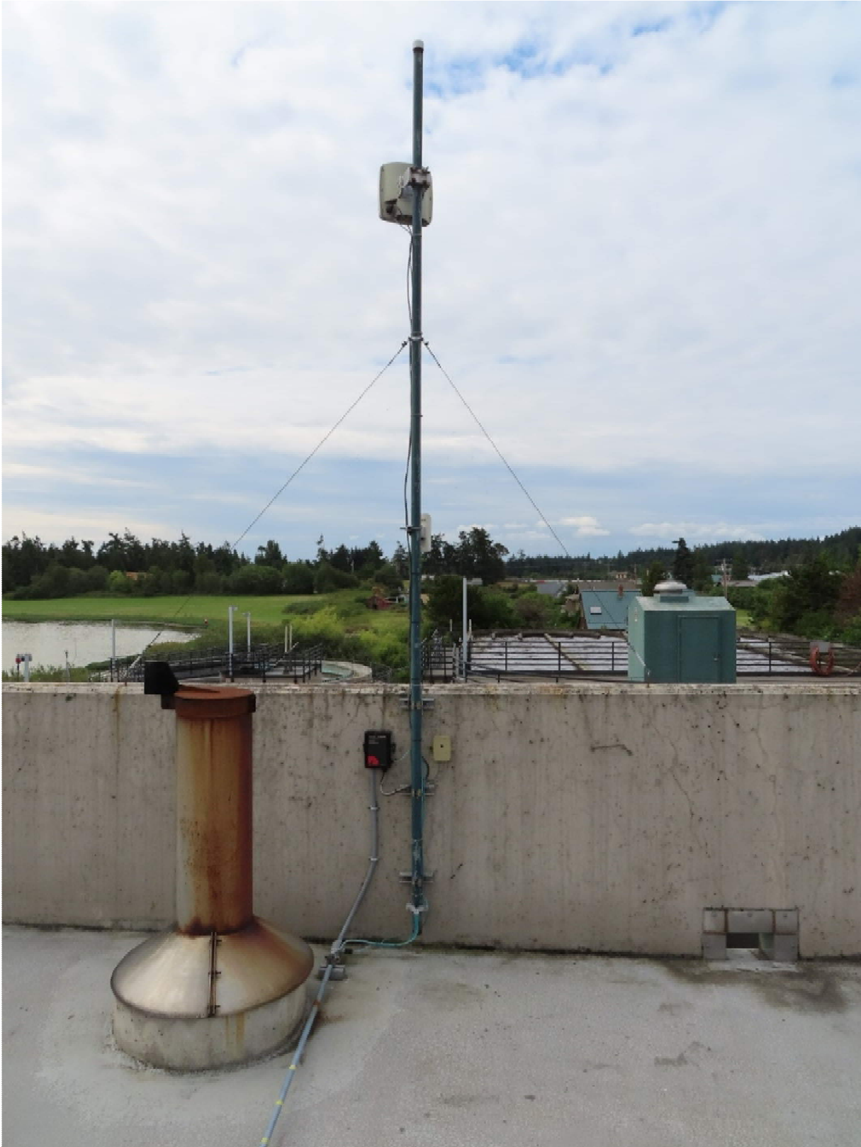
Photo 31. Abandoned network radio antenna
