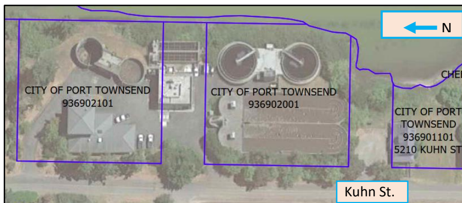
Figure 8-2 – WWTF Site Aerial
