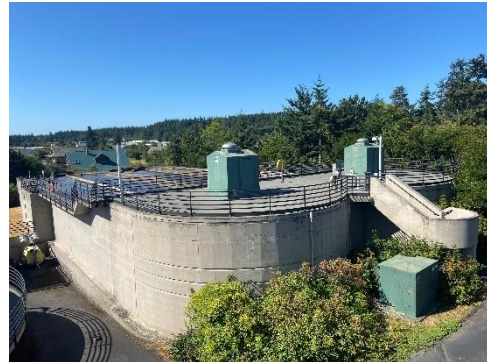
WWTF Oxidation Ditches
