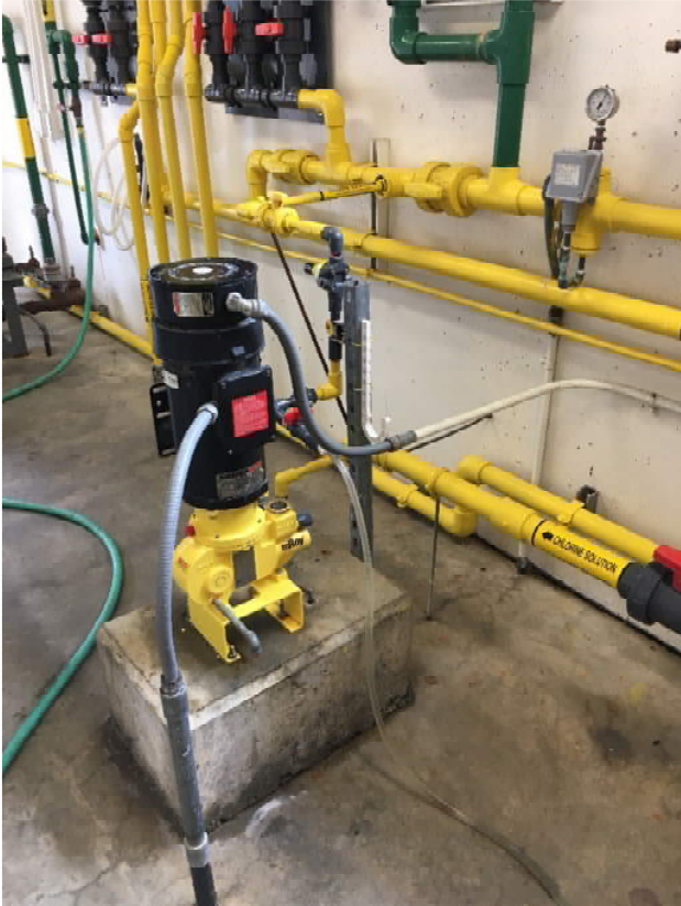
Photo 17: Hypochlorite Metering Pump
