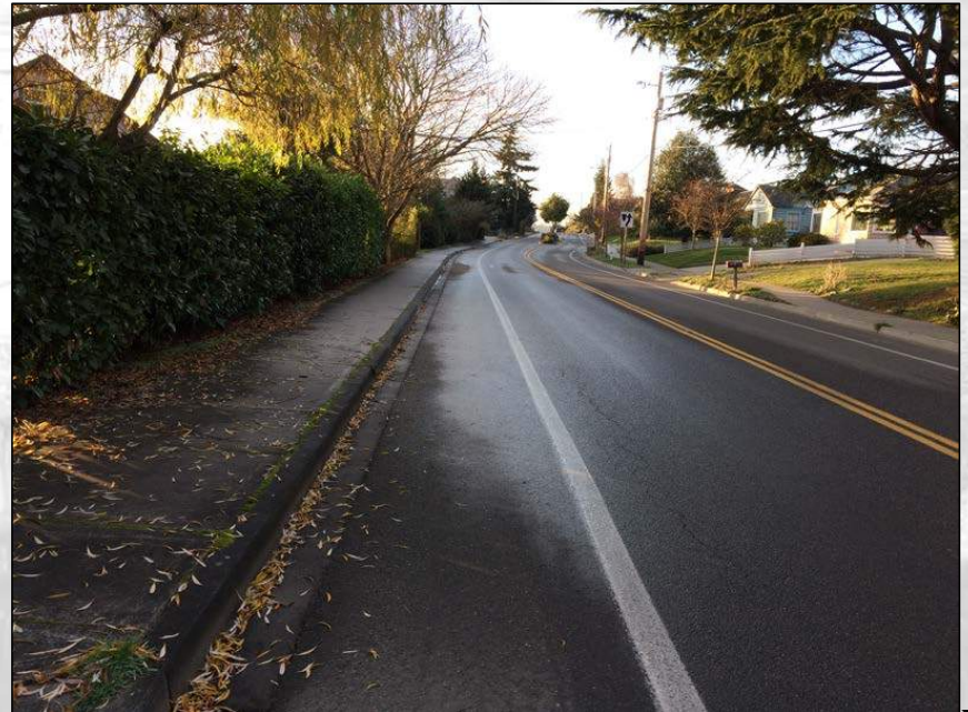
F Street – Curb and Gutter
