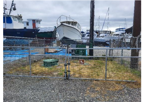
Port Lift Station
