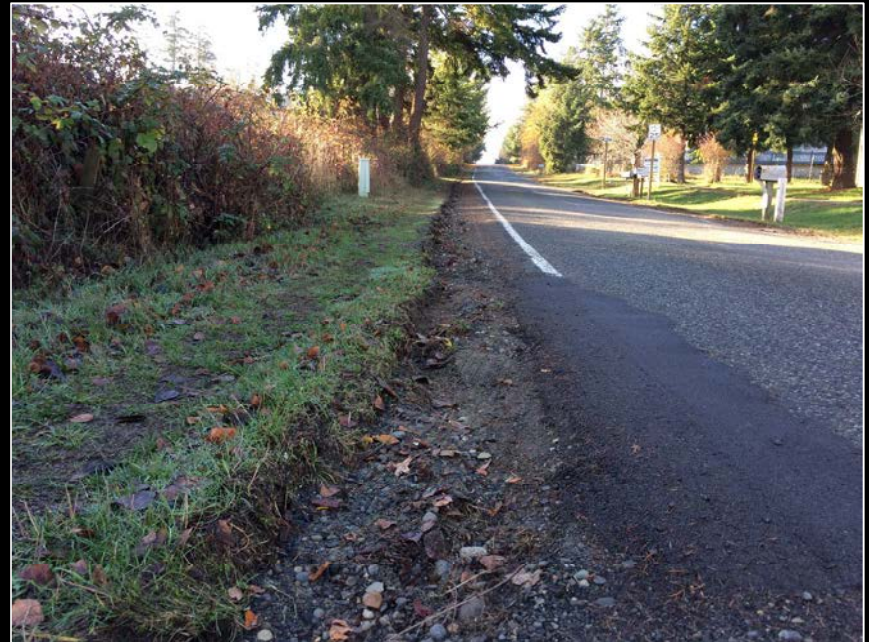
14 th Street – shoulder maintenance
