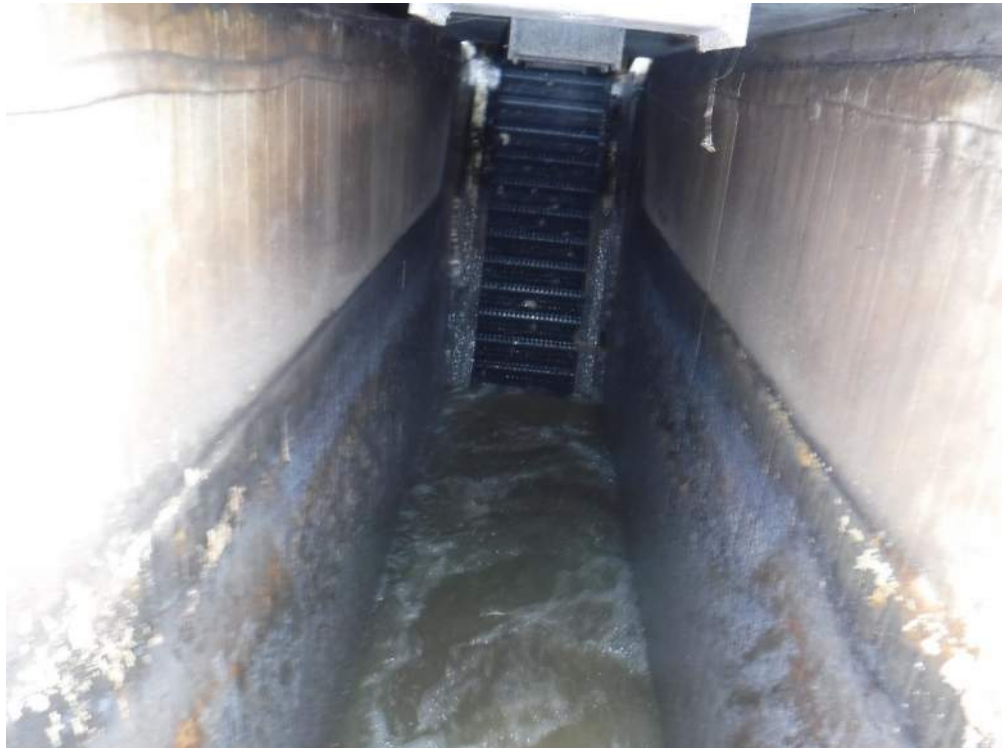
Photo 36. Traveling screen and embedded plastic liner in good condition.
