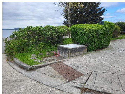
Monroe Street Lift Station
