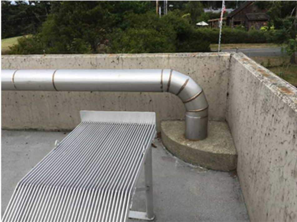
Photo 4: Manual Bar Rack
