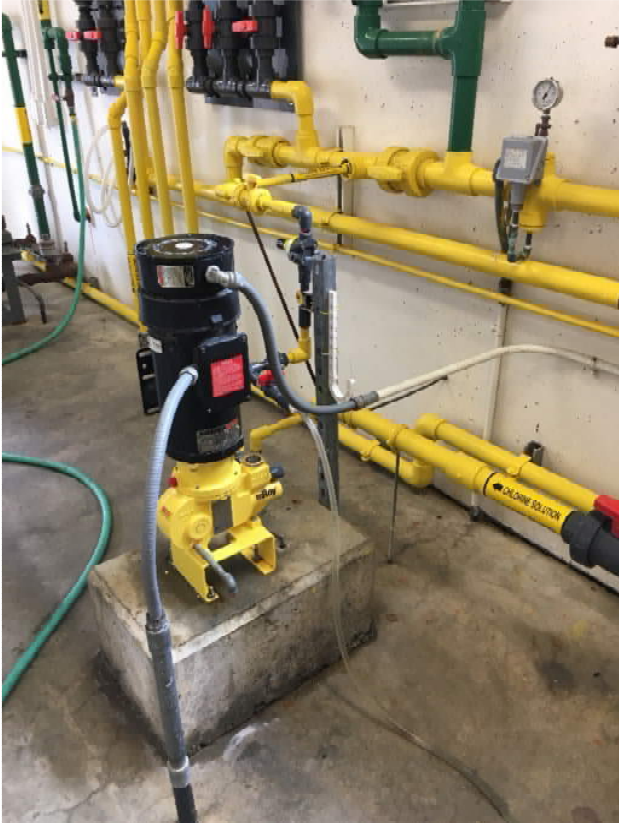
Photo 17: Hypochlorite Metering Pump
