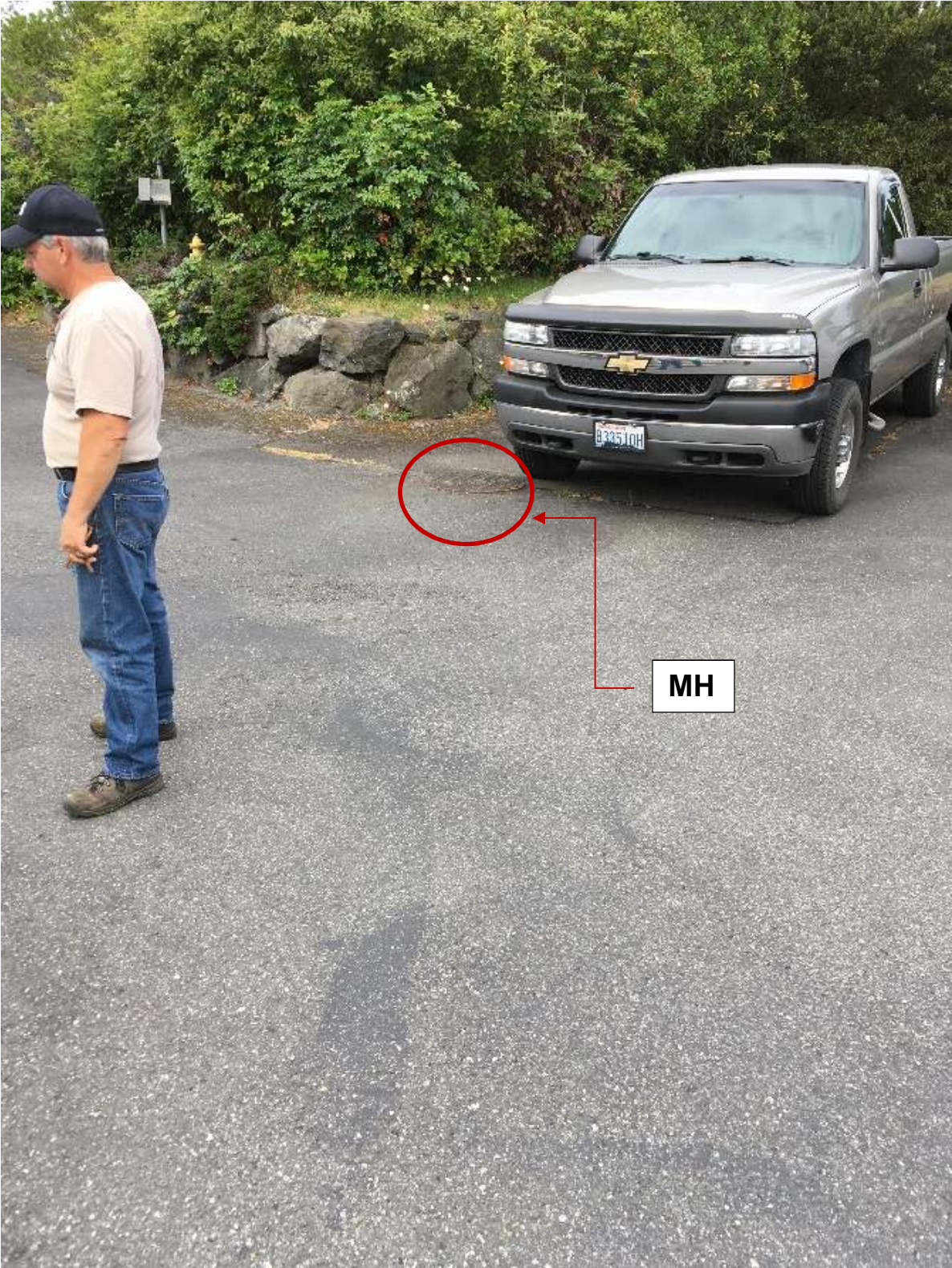
Photo 48: Potential Influent Pump Station Pump Around Manhole
