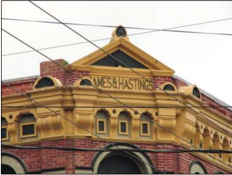
Corner sign of the James & Hastings Building November 2010. photo by Brian Moratti
