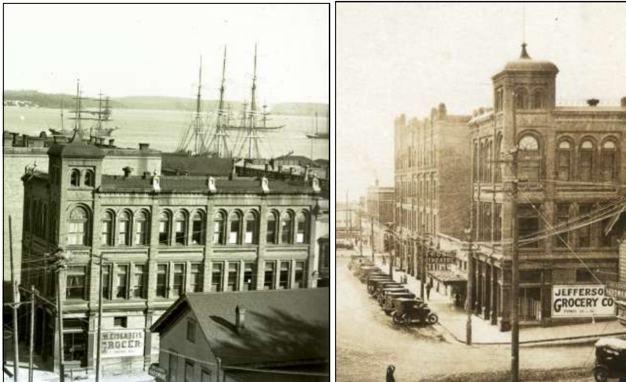
Neither of the grocery murals on the Washington Street side of the building still exist.
