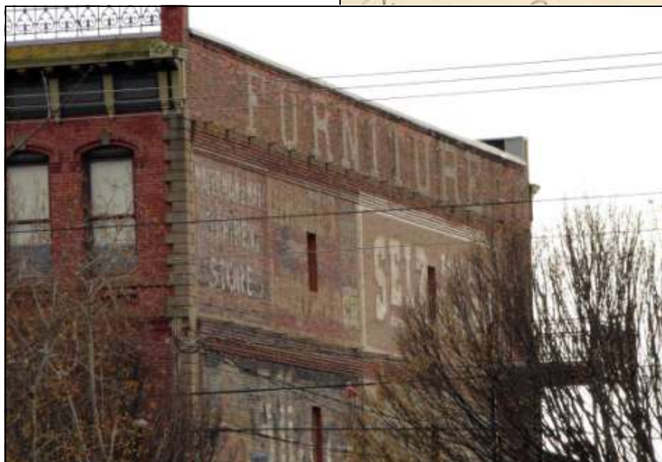
Waterman Katz Building November 2010.
