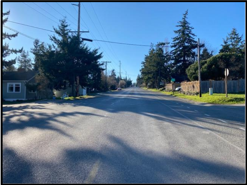
Landes Intersection Looking West & Uphill
