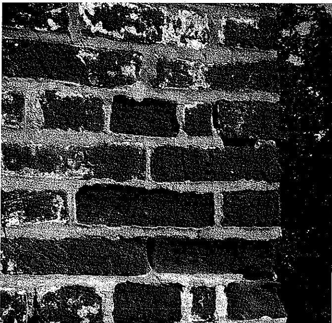
Figure 5. The use of hard, portland-cement mortar that is less permeable than the soft bricks has resulted in severe damage to this brick wall. Moisture trapped in the wall was unable to evaporate through the mortar which is intended to be sacrificial, and thus protect the bricks. As a result the moisture remained in the walls until water pressure eventually popped the surface off the bricks. Photo: National Park Service Files.
