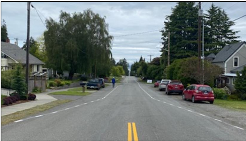
Blaine Street after temporary installation
