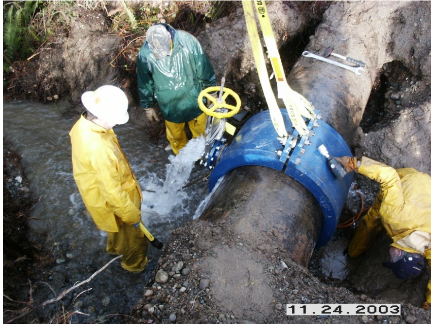
Waterline Live Repair in 2003
