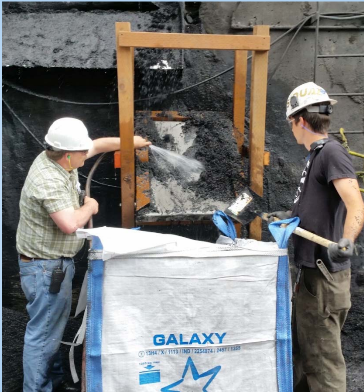
Simple trial system to rinse fines out of biochar
