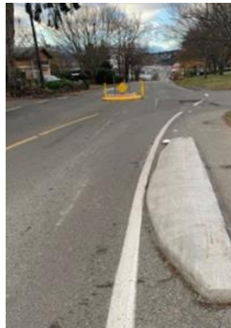
Traffic Calming Island Washington St.
