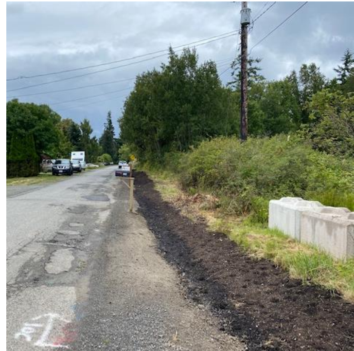
Ditching performed to fix drainage ahead of paving of Hancock Street
