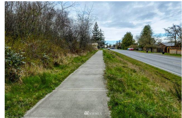
Landes Sidewalk Project
