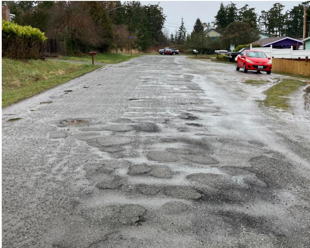
Typical Port Townsend Street Condition
