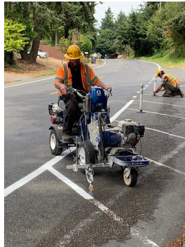
City Crews - Detail work
