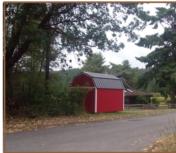
Shed constructed illegally in the public right-of-way.
