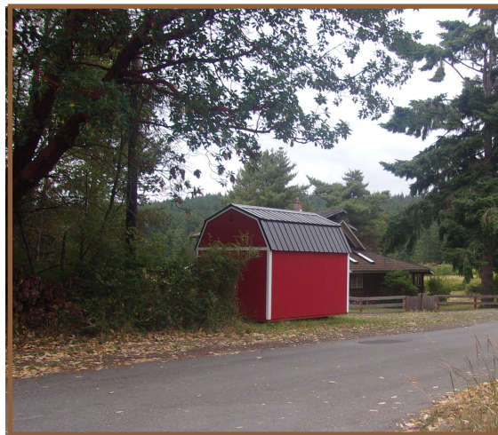
Shed constructed illegally in the public right-of-way.
