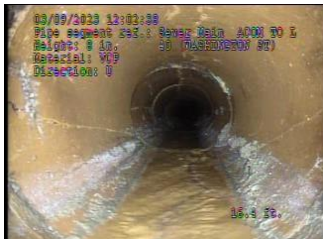
Figure 6-8 – Washington Street Sewer with Cracks
