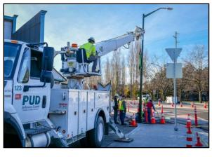
the pole. Then the pole will be set in place with a derrick digger. Each streetlight placement is unique, but typically it takes about four hours to install a streetlight including wiring. Once installed, the streetlights will immediately be energized and ready for service. If you observe a streetlight is out, please call the PUD's main number at 360-385-5800.
