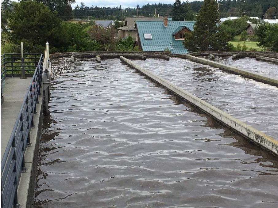
Photo 9: Oxidation Ditches
