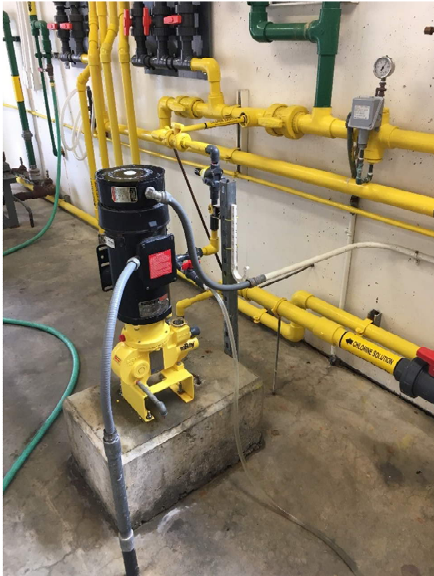
Photo 17: Hypochlorite Metering Pump
