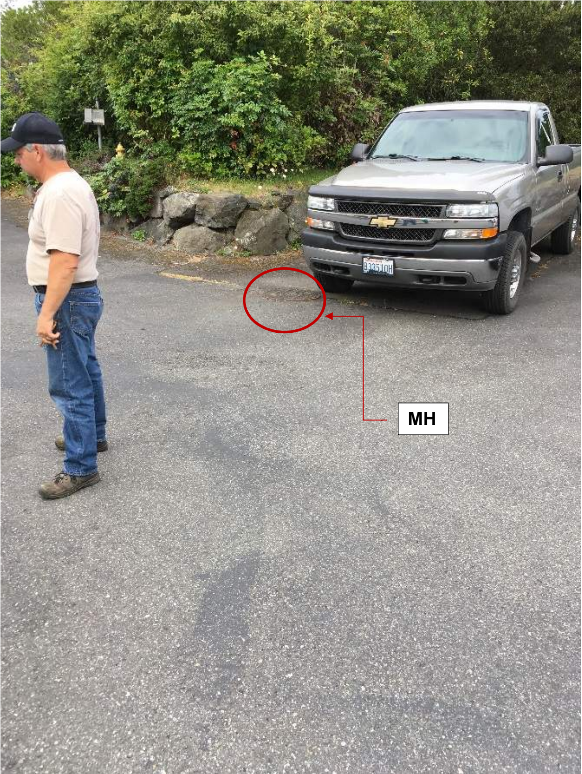
Photo 48: Potential Influent Pump Station Pump Around Manhole
