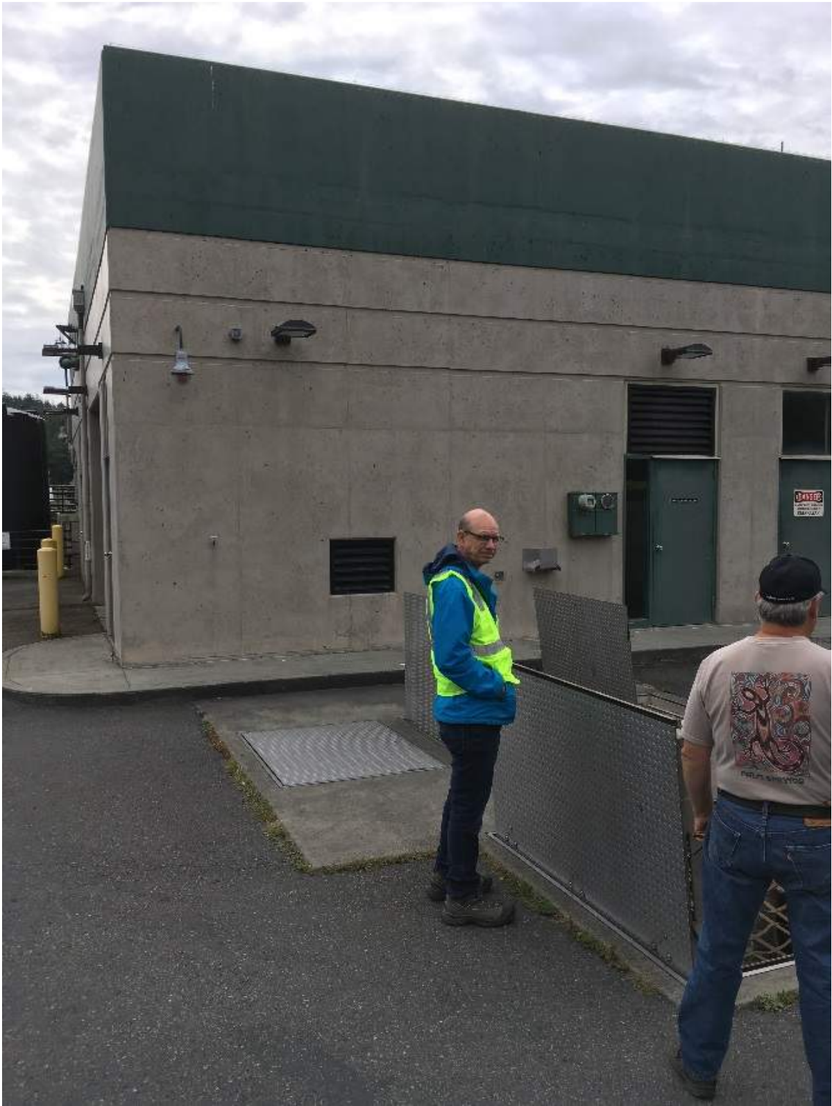
Photo 49: Influent Pump Station Pump Around Discharge to Pass Over Building Parapet
