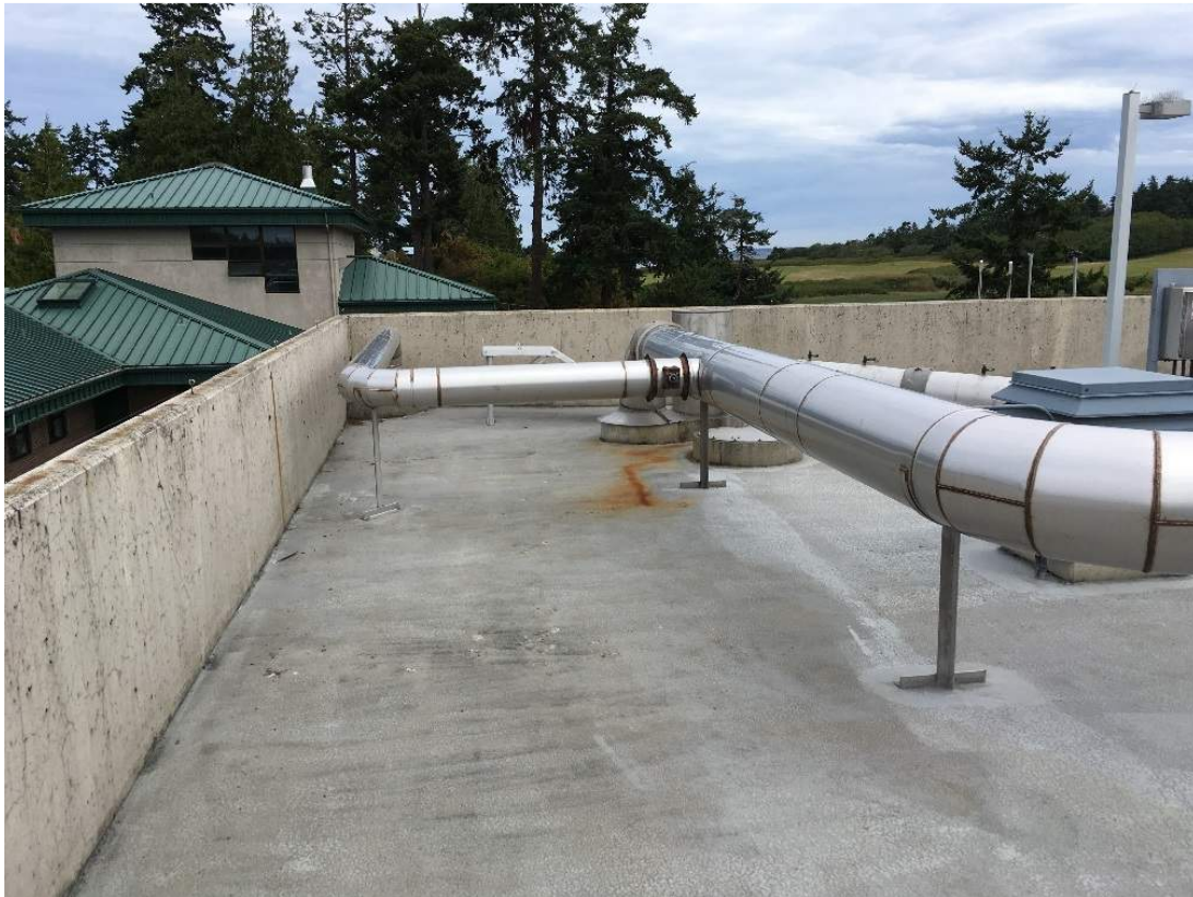
Photo 50: Route of Pump Around Over Parapet to Channel Upstream of Bar Screen and Odor Control Duct Down to Influent Pump Station.
