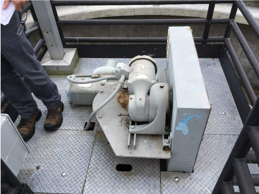
Photo 13: Clarifier Drive Mechanism
