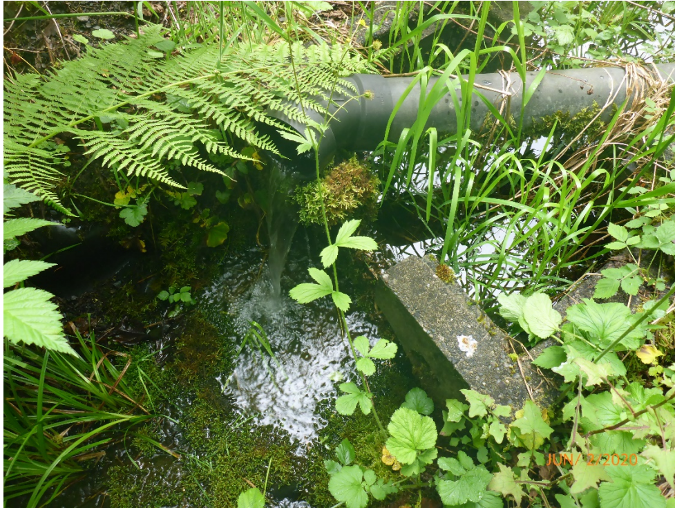
Photo 1: Weir and drain pipe at downstream toe area of North Dam.
