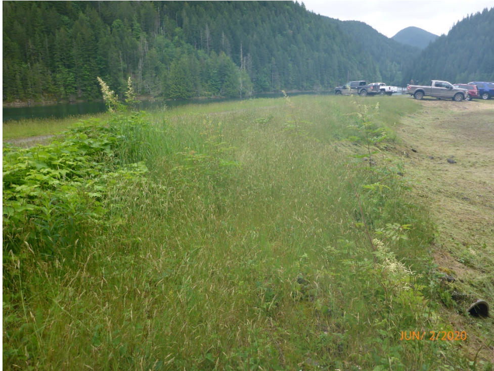
Photo 5: Southern saddle section of East Dam.
