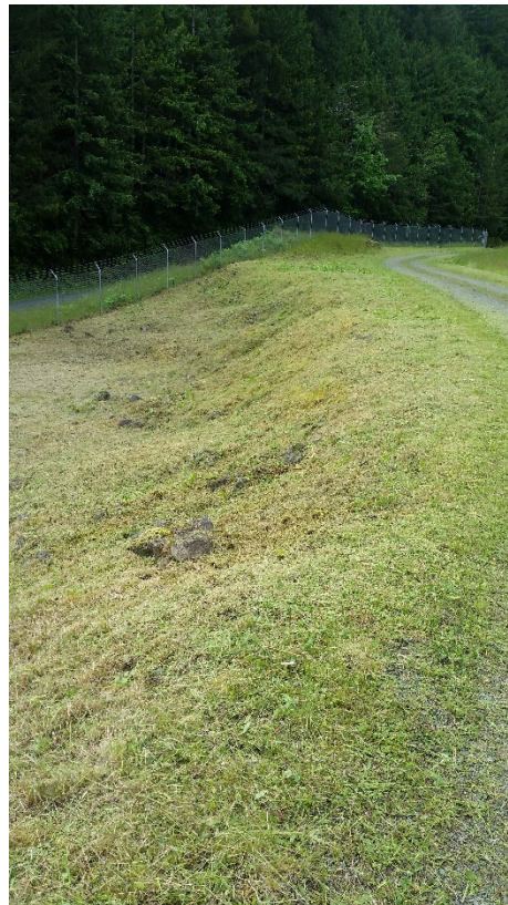
Photo 6: Southern saddle section of East Dam cleared of vegetation after inspection.
