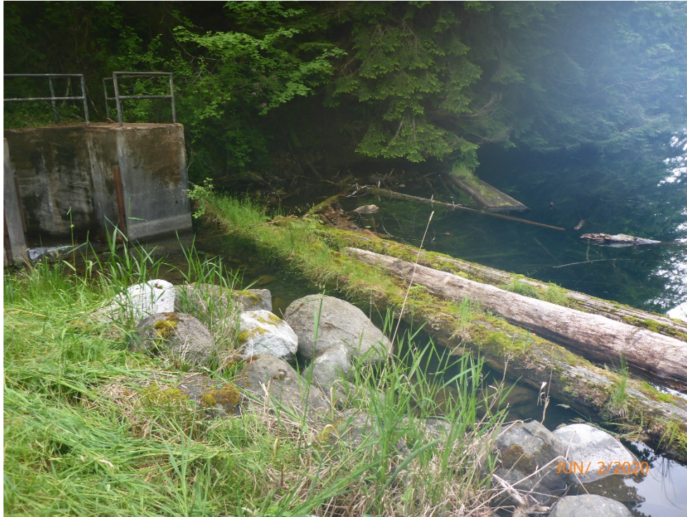
Photo 9: Spillway entrance channel at North Dam.
