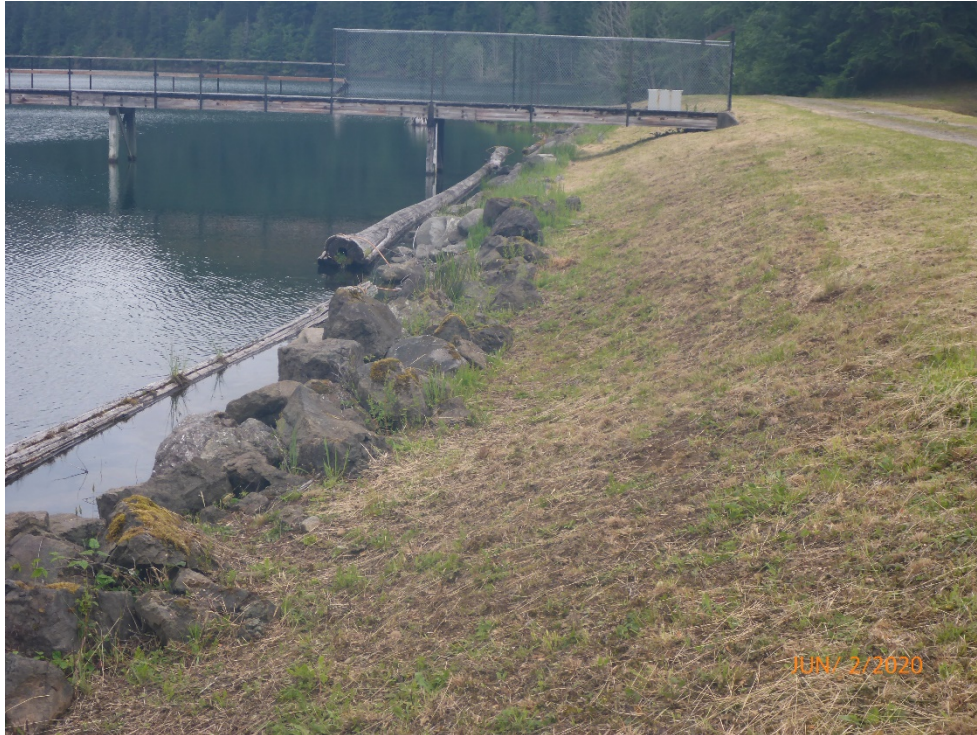
Photo 3: Upstream slope at East Dam.
