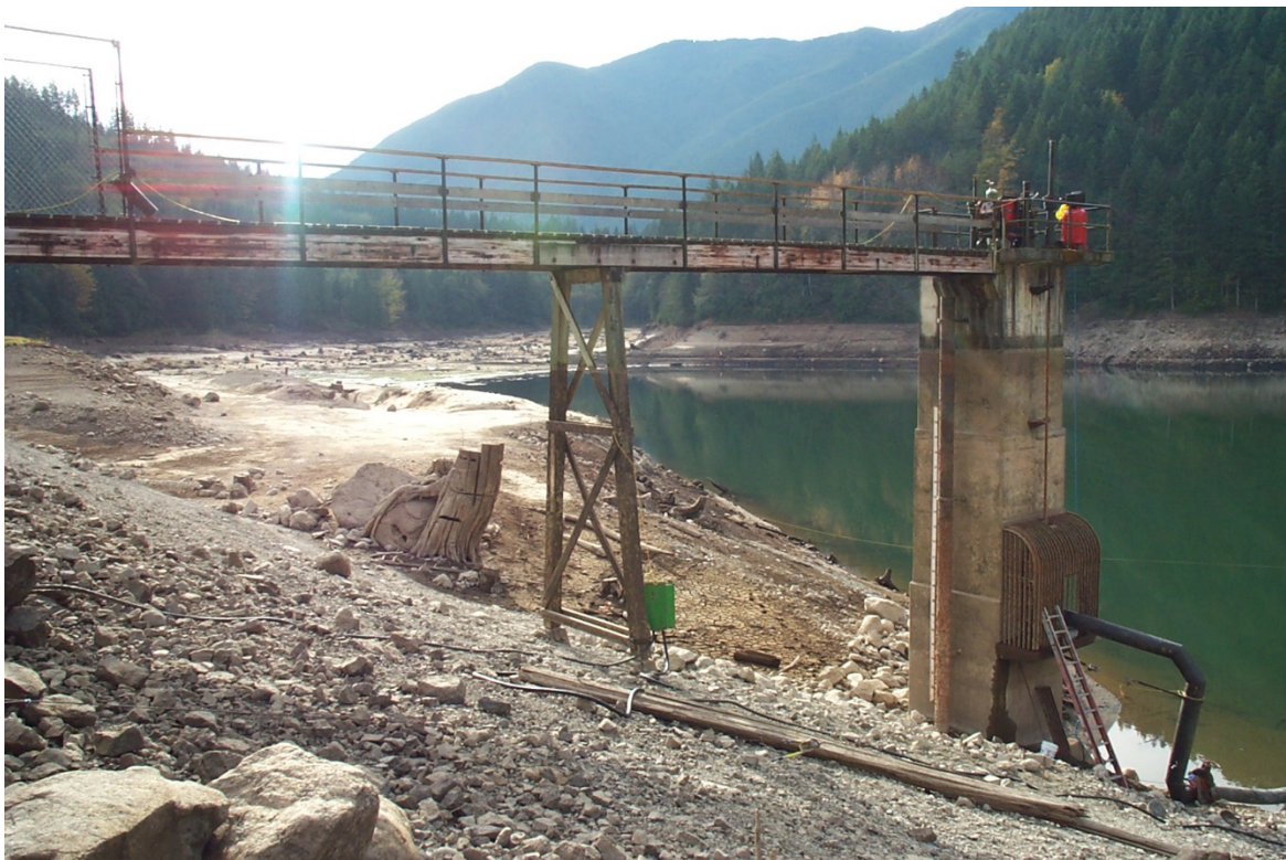
Photo 4: Upstream slope at East Dam (October 2002).
