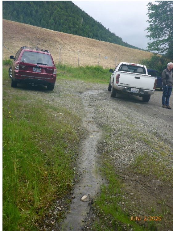
Photo 7: Seepage area on downstream foundation area at East Dam.
