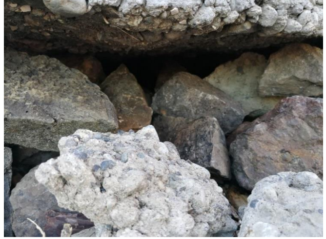
B. Foundation rocks underlying concrete pathway
