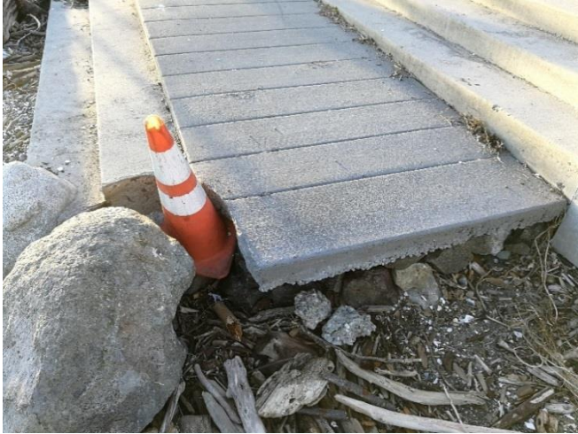
A. Concrete pathway for wheelchair and beach access
