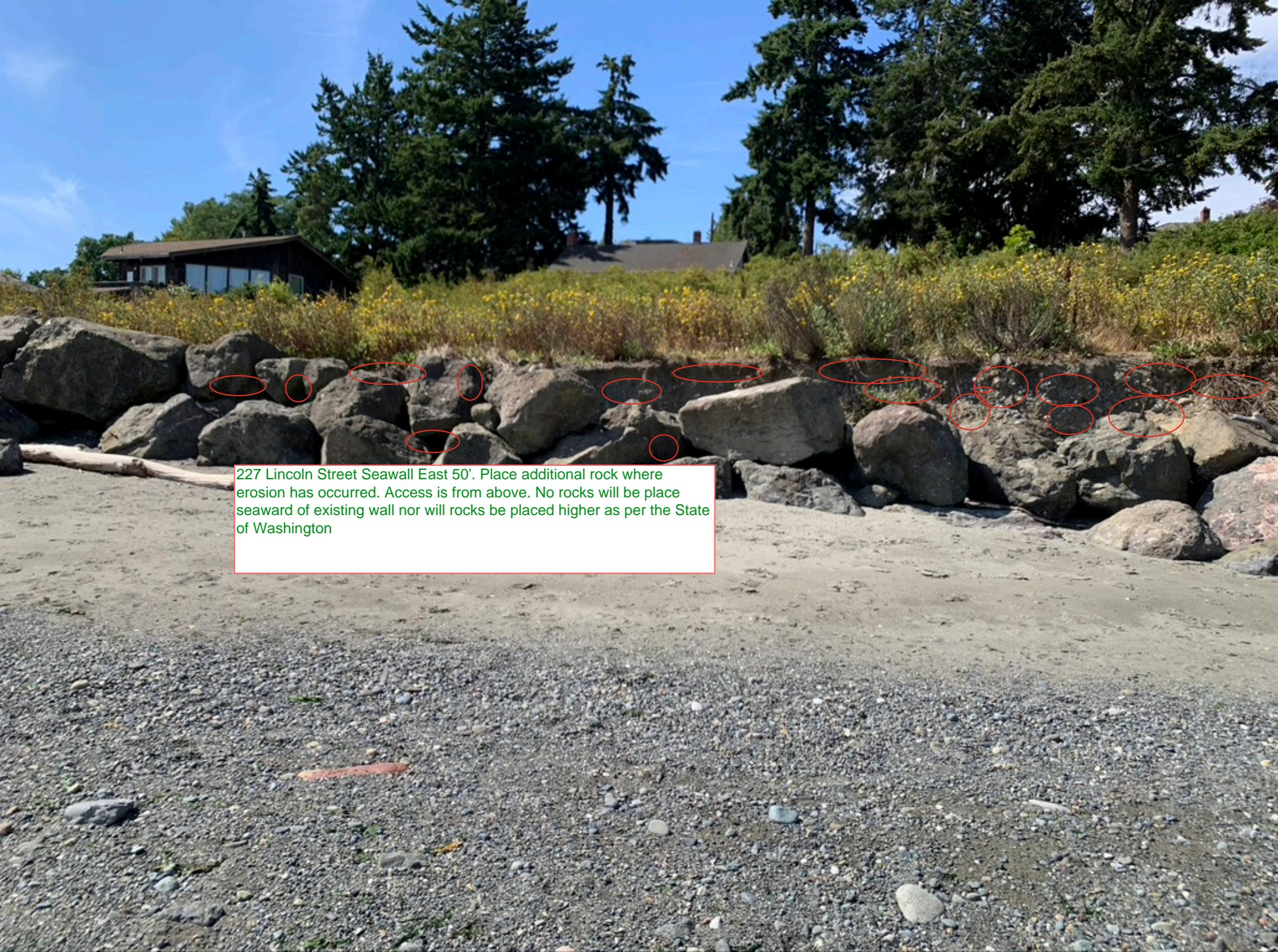
227 Lincoln Street Seawall East 50'. Place additional rock where erosion has occurred. Access is from above. No rocks will be place seaward of existing wall nor will rocks be placed higher as per the State of Washington
