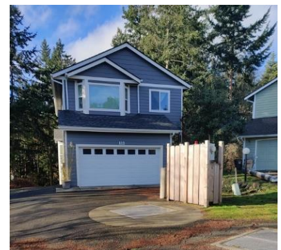
Island Vista Lift Station
