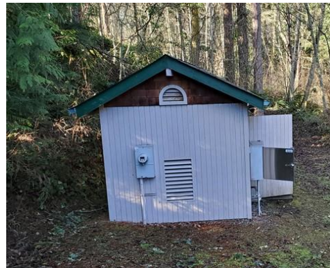
Hamilton Heights Lift Station
