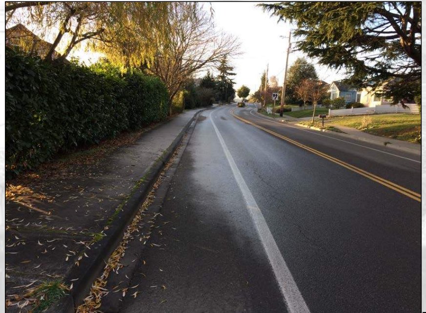
F Street – Curb and Gutter
