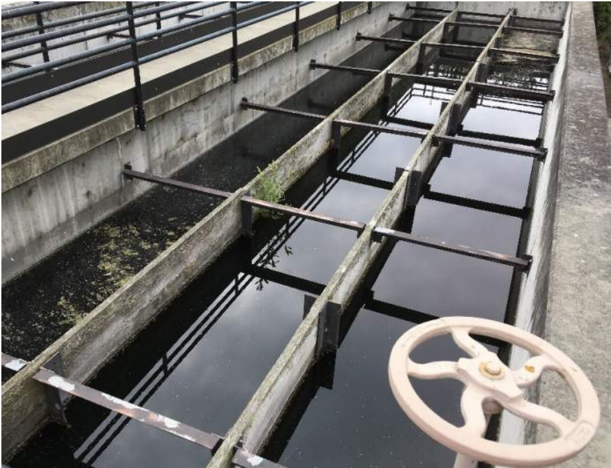
Photo 15: Chlorine Contact Basin
