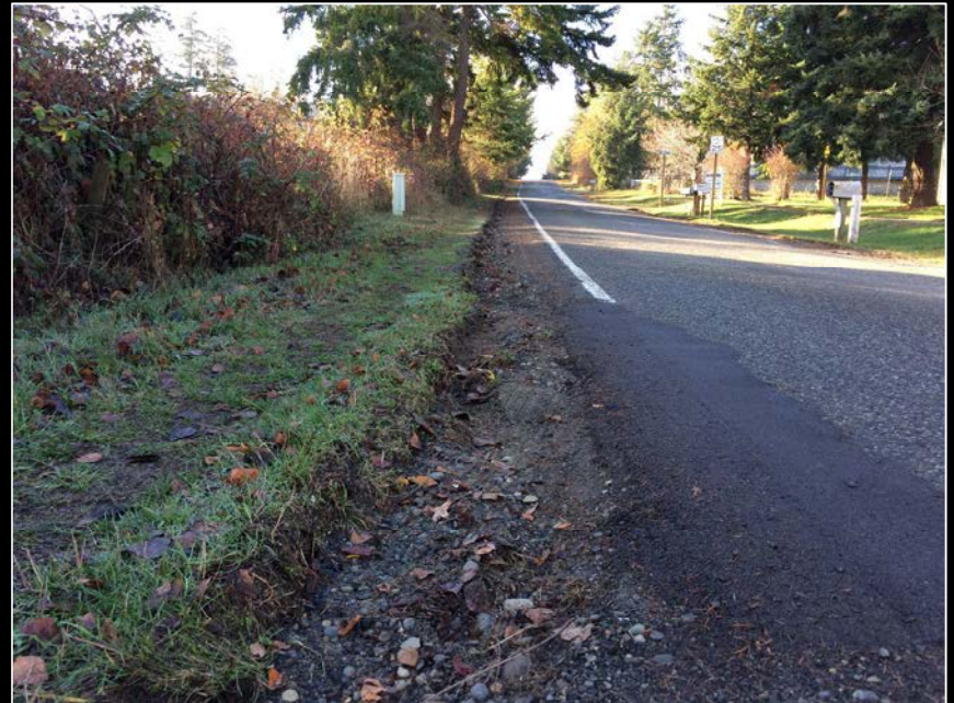
14 th Street – shoulder maintenance
