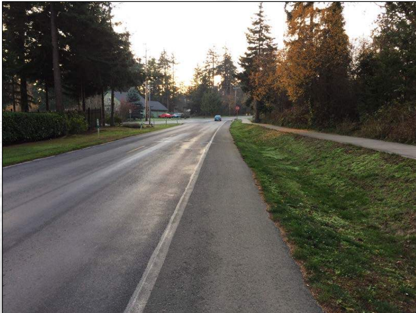
Discovery Road – Road side Swale
