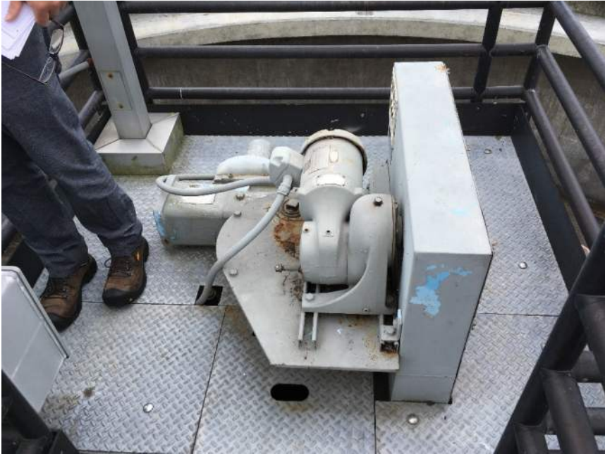
Photo 13: Clarifier Drive Mechanism
