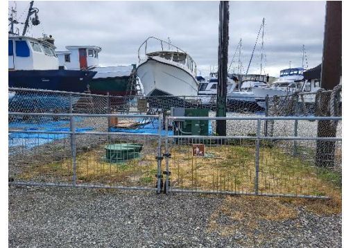
Port Lift Station
