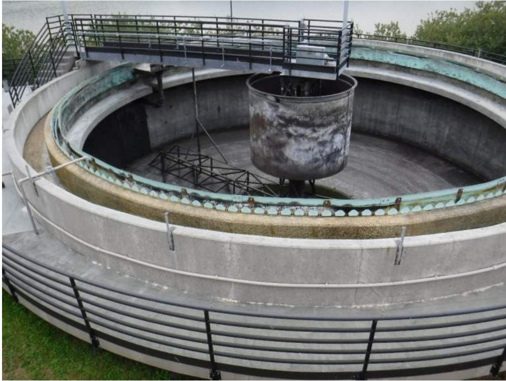
Photo 44. South secondary clarifier, empty at the time of inspection.
