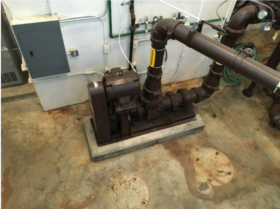
Photo 19: Belt Press Feed Pump
