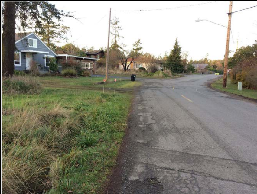
Sheridan Street – Swales needed
