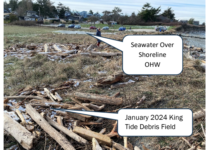
2024 King Tide Debris Field Overtopping Shoreline
