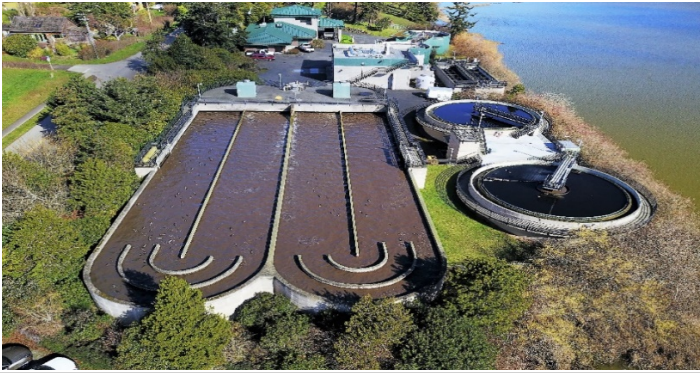
Aerial looking at Wastewater Treatment Plant (WWTP)
