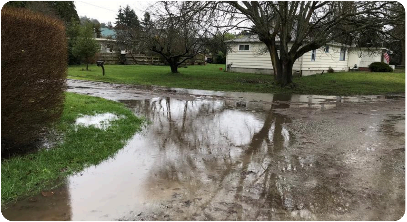
Drainage issues along Pacific and Milo Streets.
