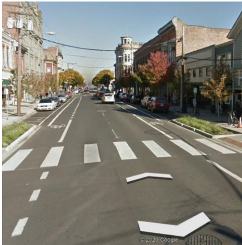
Water Street Lane Constriction
