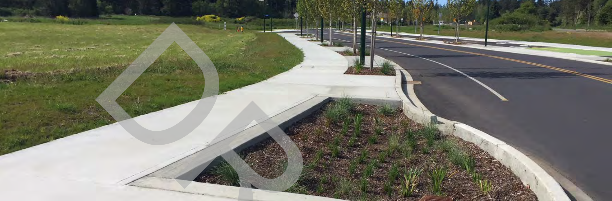
Bioretention facilities along Rainier Street (Source:AHBL)
