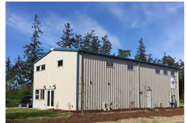
New brewery within the Port Townsend Business Park
