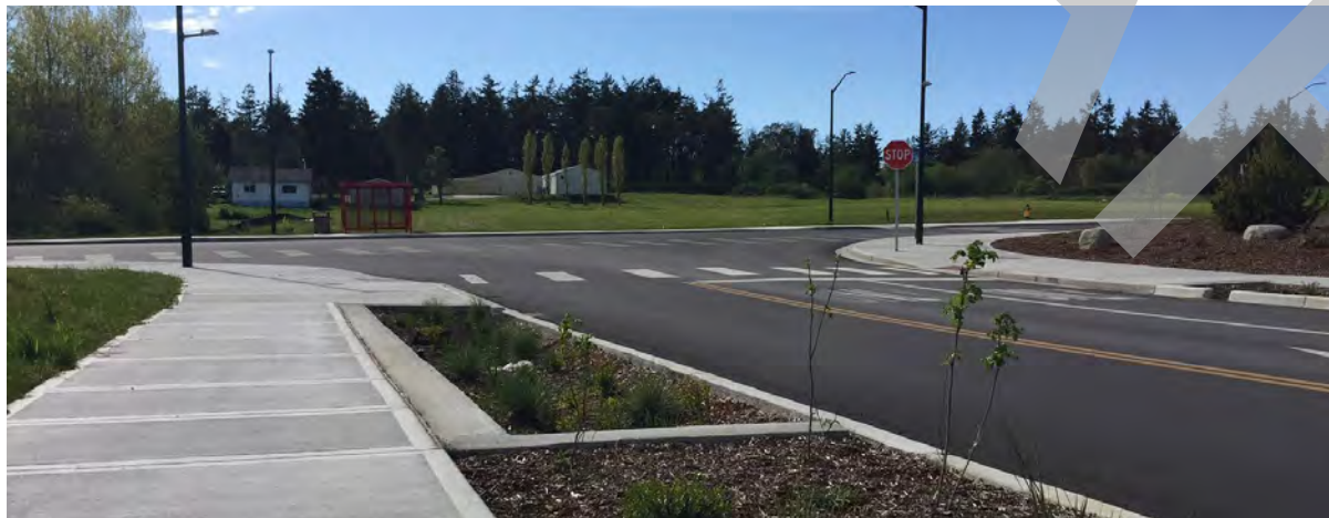
Rainier Street designed for multimodal transportation and green stormwater management.
