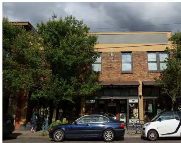
Street design that serves a variety of users including vehicles, bicyclists, and pedestrians.
