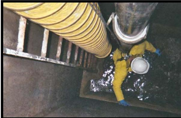
Employees risk their lives to enter a confined space and remove grease from pumping stations. The individual above needed to be extracted from the confined space due to a change in air quality.
